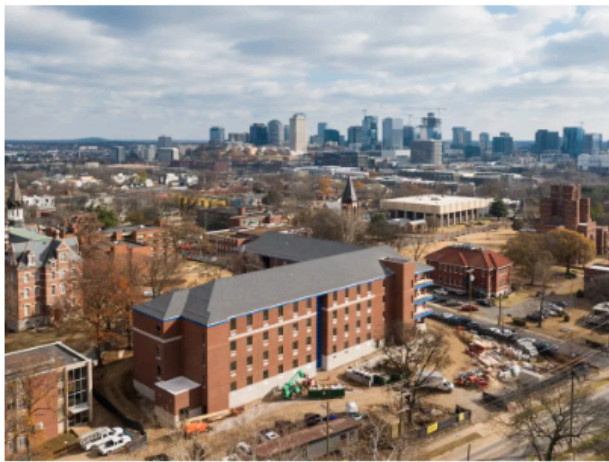
In addition to working on research laboratories, the main library, a fitness center and the renovation of Jubilee Hall at Fisk University, Jared Bradley and his partner Scott Delano's construction company Certified Construction Services is currently building a new on-campus residential hall. Photo by Ford Photographs, courtesy of The Bradley Projects
