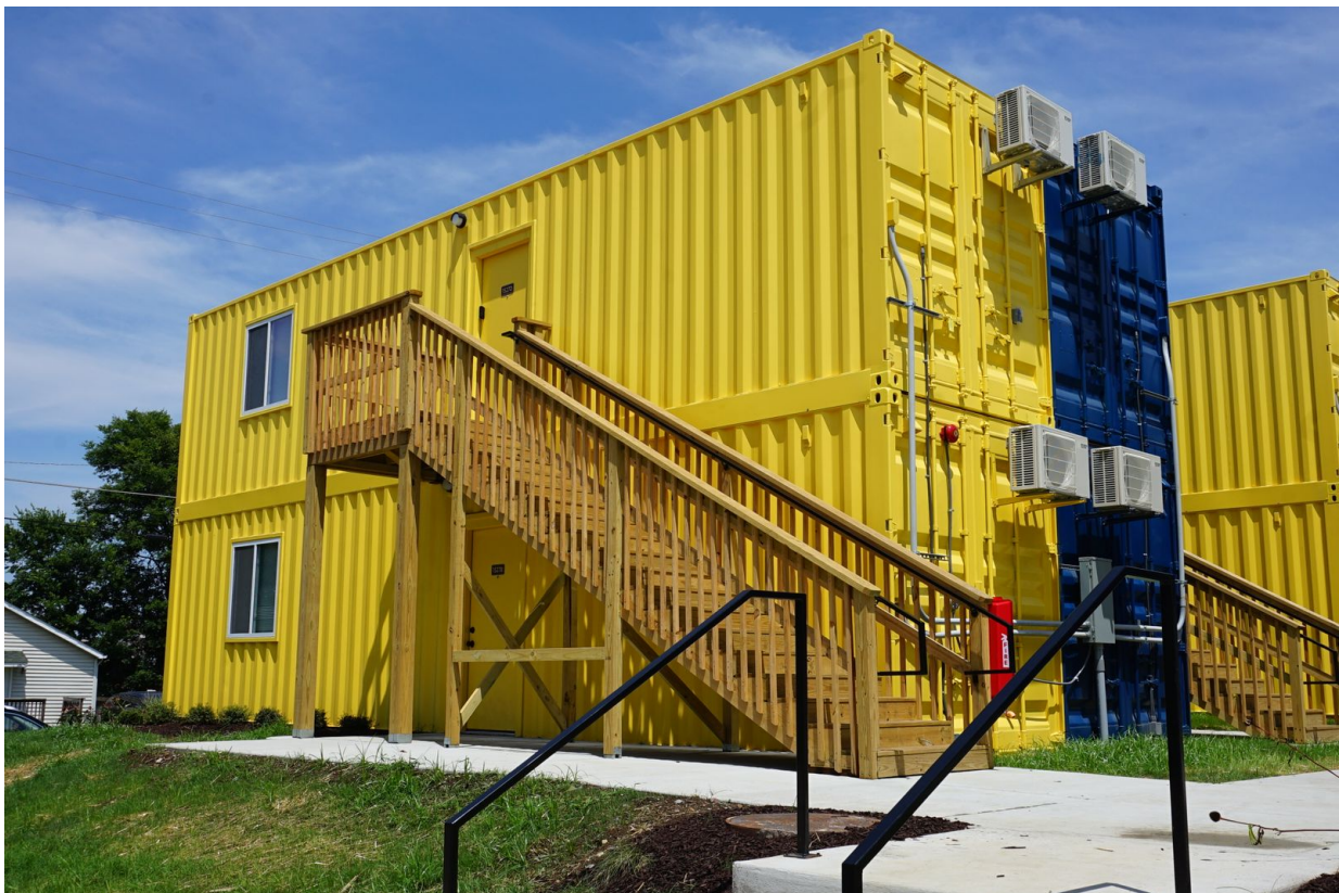
The entrances to the shipping container dorms at Fisk University. The units were designed to meet the school's housing needs while another dormitory is under construction.
